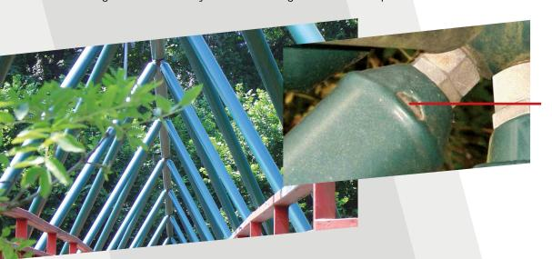
No under-film corrosion after years of exposure.
