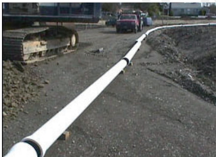
Harbour Island, Seattle, pipe coated in PPA 571
