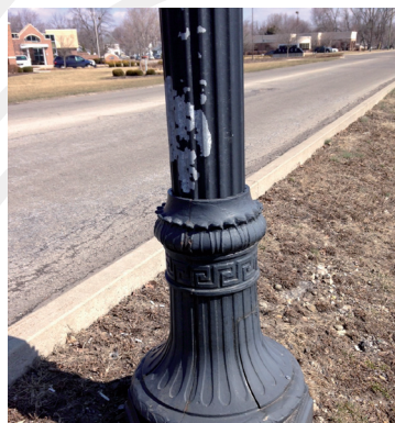
The polyester coating has failed
