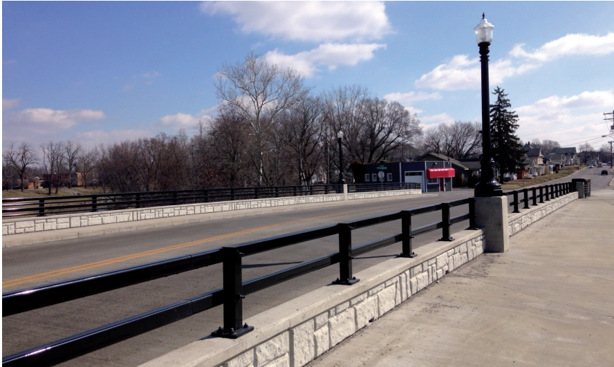
Jackson Bridge, Muncie, Indiana; Railings and columns coated in Plascoat PPA 571
