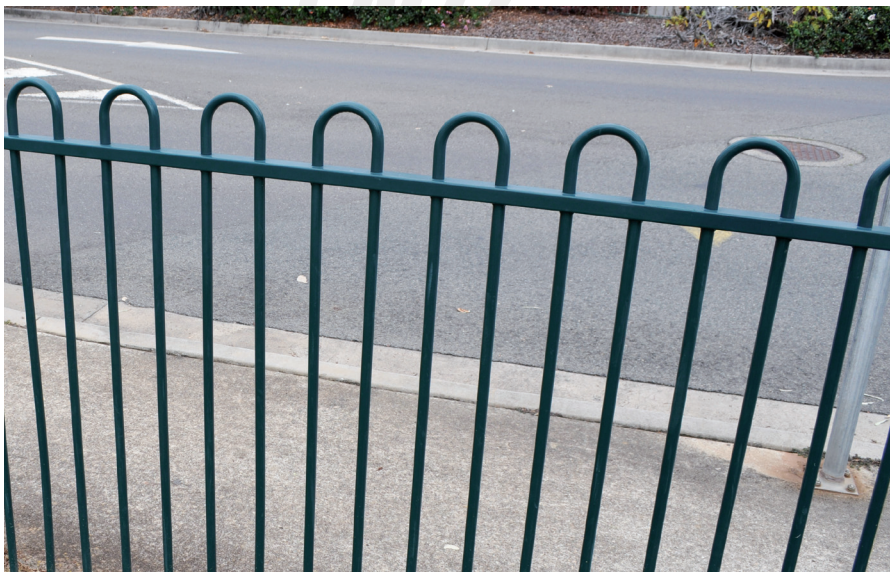
In this recent photograph, after twenty years by the sea, the Plascoat PPA 571 coated fence is still in excellent functional and cosmetic condition.
