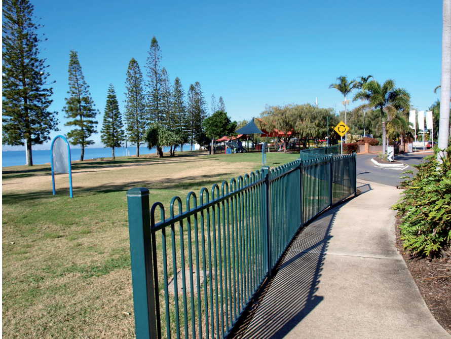
This ornamental fence is coated in Plascoat PPA 571.
