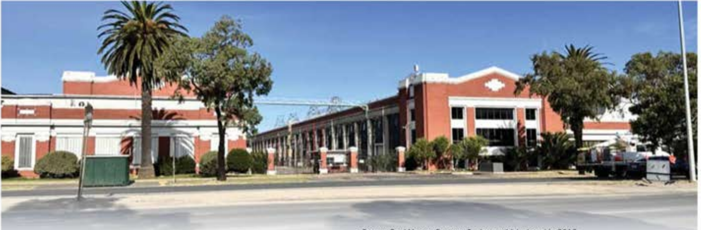
Former Ford Motors Factory, Geelong, which closed in 2016. Credit S. Cooke. www.mdpi.com/2571-9408/6/3/162
